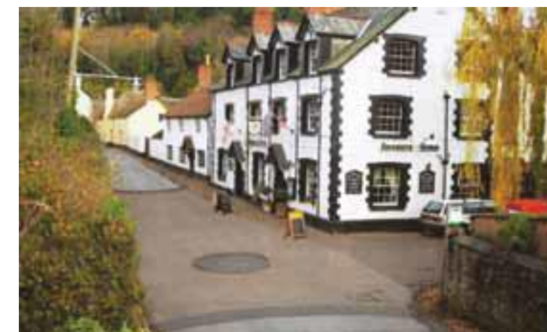
Figure 184 Dunster, Exmoor – showing how simple footpath realignment, surface materials and removal of signs and lines can create a very different lower speed environment that emphasises the character of the place. Images from Hamilton Baillie.
