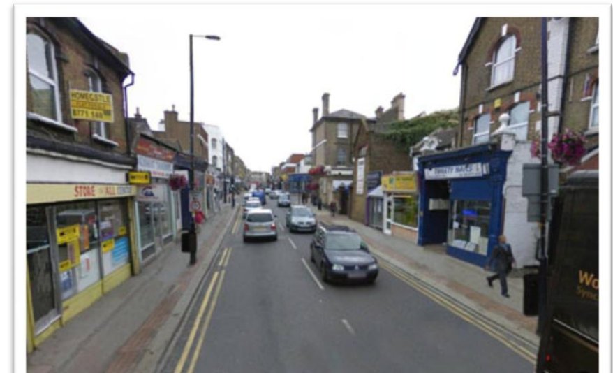
Figure 125 Step 3-Merging functions involves maximising the effectiveness of street furniture required. Bins are lifted from the ground and attached to existing lamp columns, which also accommodate new hanging flower baskets.
