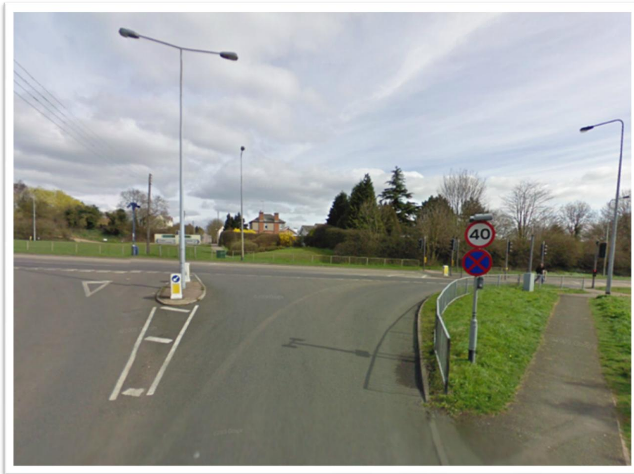
Figure 106 The A6 acts as barrier to pedestrian movement. Pedestrian guard rails mean that pedestrians are pushed off the most direct route across the road.
