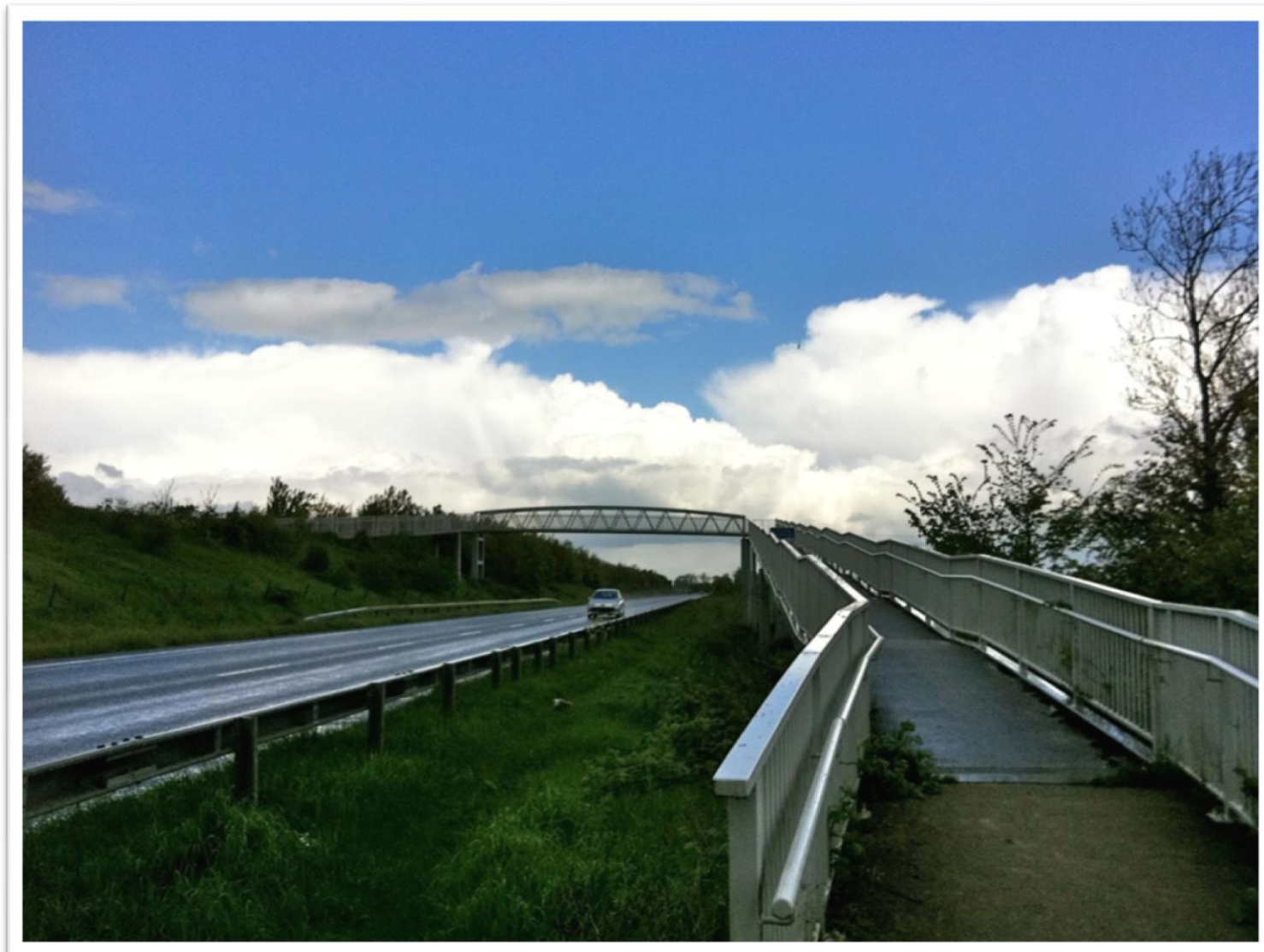
Figure 120 Pedestrian bridge over A6 Image courtesy of Jo Miles
