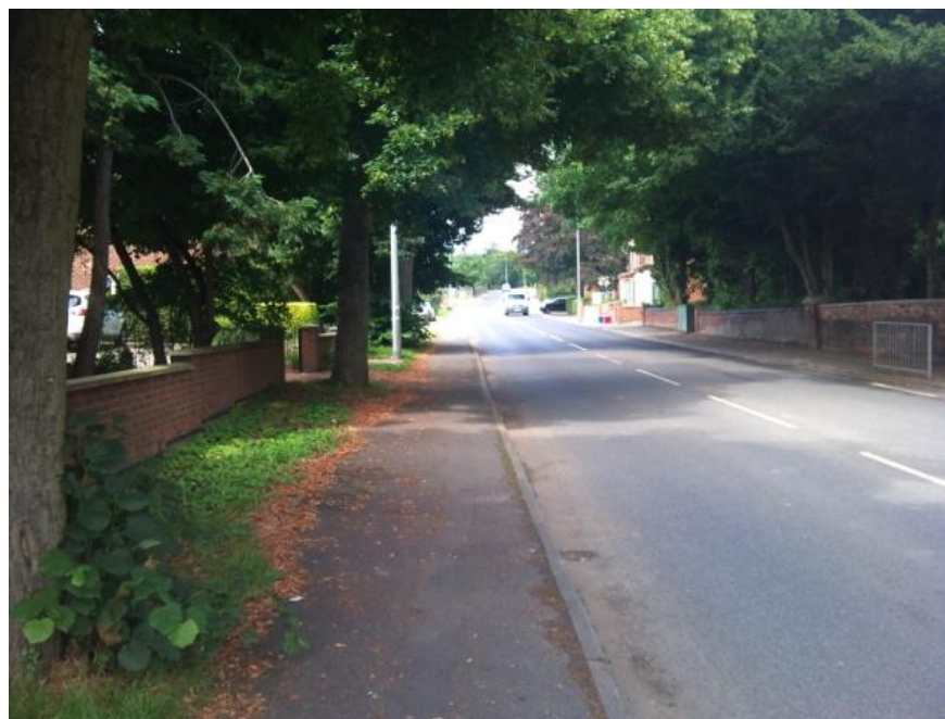
Figure 183 Harborough Road – simple measures to visually narrow the road to help slow speeds, different surface treatments and wider pavements to prioritise walking and cycling movement on this key radial. Good ideas are to be found in the Hamilton Baillie Associates “Traffic in Villages” toolkit for rural communities http://www.hamilton-baillie.co.uk/files/publications/50-1.pdf
