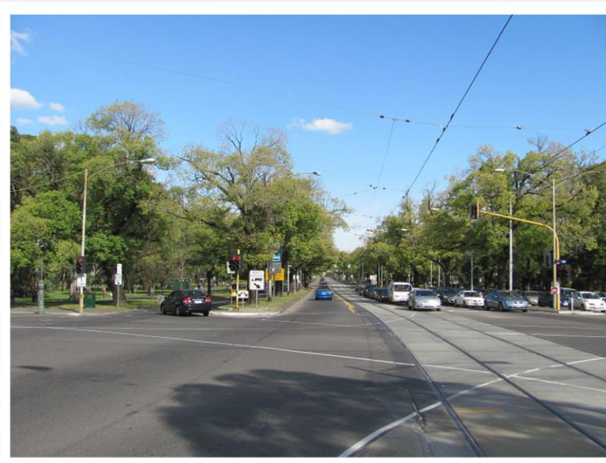
Figure 39 Multi lane, high traffic route with 4 main carriageway lanes, and 2 side streets, wide pavements, tree planting, central tree planted median – Royal Parade, Melbourne shows a major traffic flow road can still be easy to cross and pleasant for pedestrians. Image Copyright of Orderinchaos
