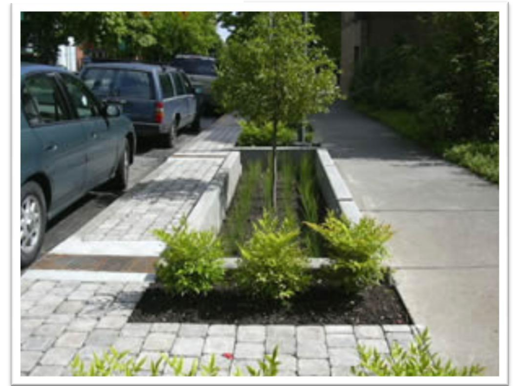
Figure 67 Storm water planter and landscaping build out on 12th Avenue, Portland (Image courtesy of City of Portland)
