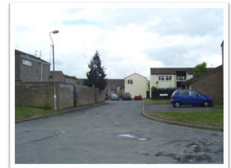
Figure 46 Radburn estate. Photo JPU
