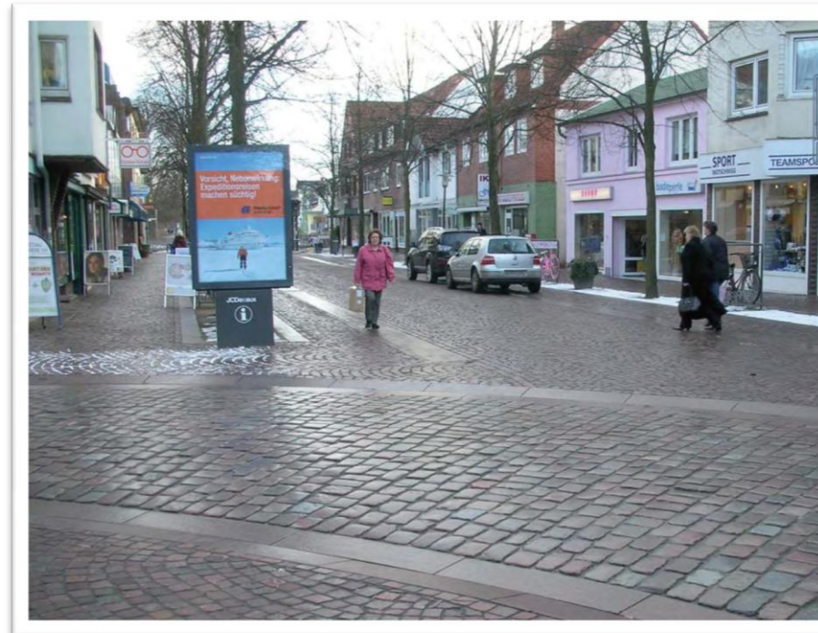
Figure 80 Ahrensburg, Germany. A simple combination of robust natural materials allows for through traffic, parking and pedestrian movement (image from Hamilton Baillie Associates)
