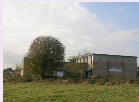
Existing Desborough Leisure Centre
