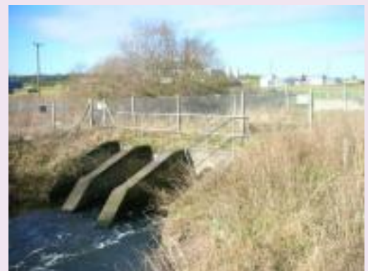
Broadholme Wastewater Treatment Plant
