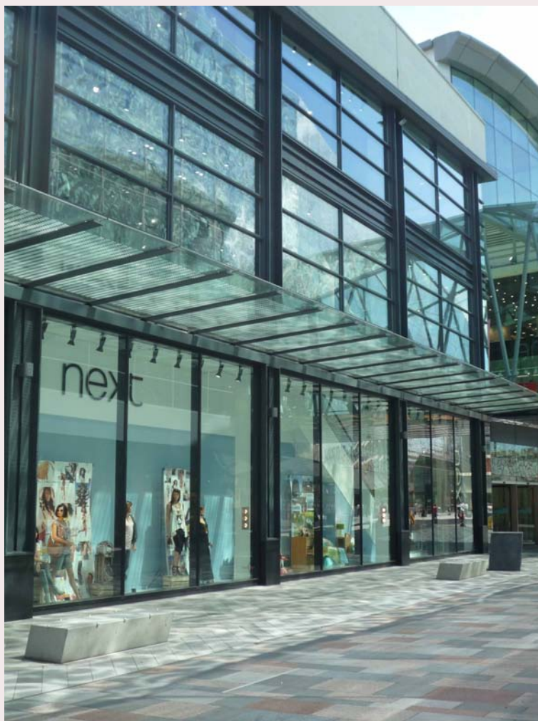
A modern shop development in Leicester with a glass canopy. Note the minimal use of signage to create an attractive unit
