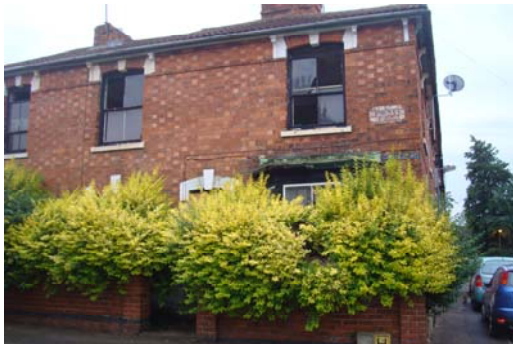
Empty property at Grange Road, Kettering (before)
