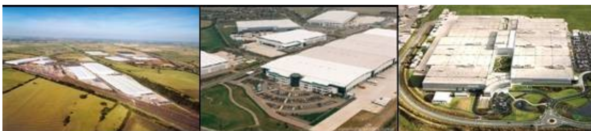
Distribution and Logistics; DIRFT, ProLogis and Hams Hall (Left to Right)
