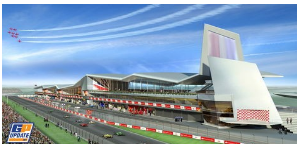
New Pit and Paddock complex (under-construction), Silverstone Northamptonshire
