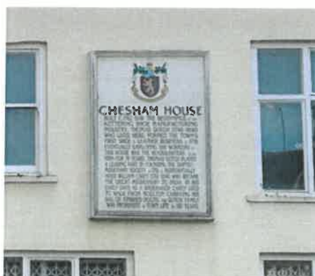
Existing plaque between first floor windows, on existing front (east) elevation
