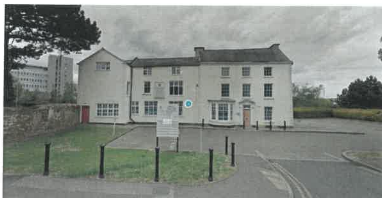
Existing front (east) elevation. Source: Google Maps
