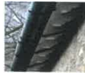
CAST IRON CAST HALF ROUNDED GUTTERS ON RAFTER BRACKETS, BEYOND DOWNPIPES, RECTANGULAR HOPPERS
