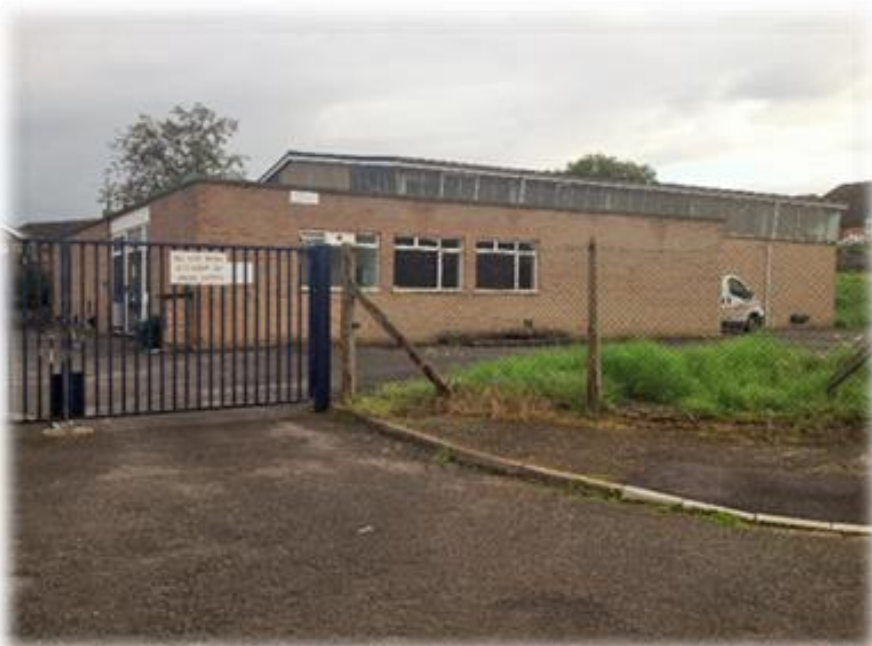
The existing BT Exchange in Church Street
