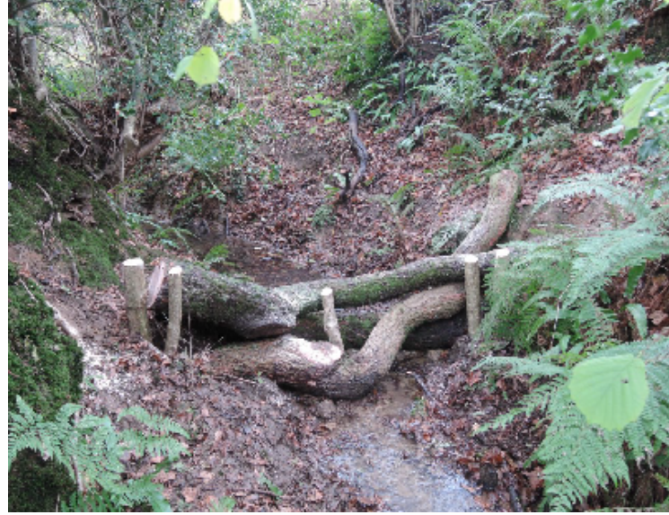
Leaky Dam (FWAG Southwest, 2016)
