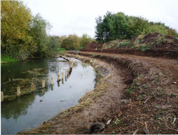
Two-Stage channel under construction (RNRP, 2015)
