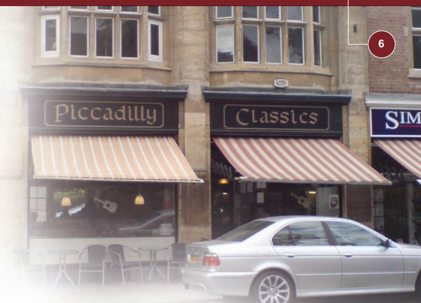
Piccadilly Buildings: A good example of shopfront, signage and awning
